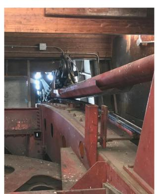
Damage at Top Terminal, Carrier Carriage and Buffer
