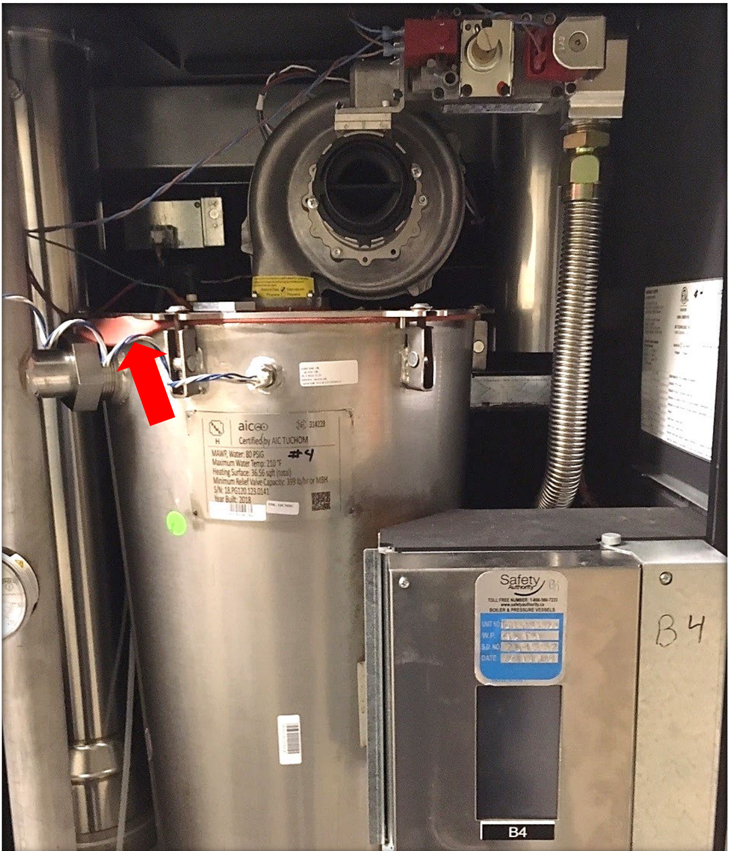
Image 7 – Pressure vessel gasket blown out from delayed ignition on Boiler 4 (example 3 of 4)
