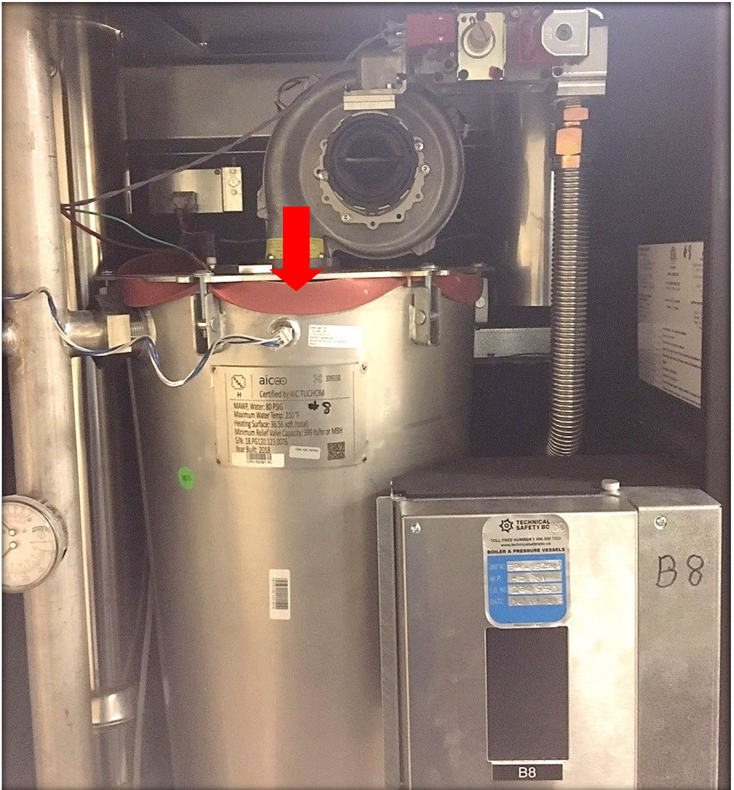
Image 5 – Pressure vessel gasket blown out from delayed ignition on Boiler 8 (example 1 of 4)
