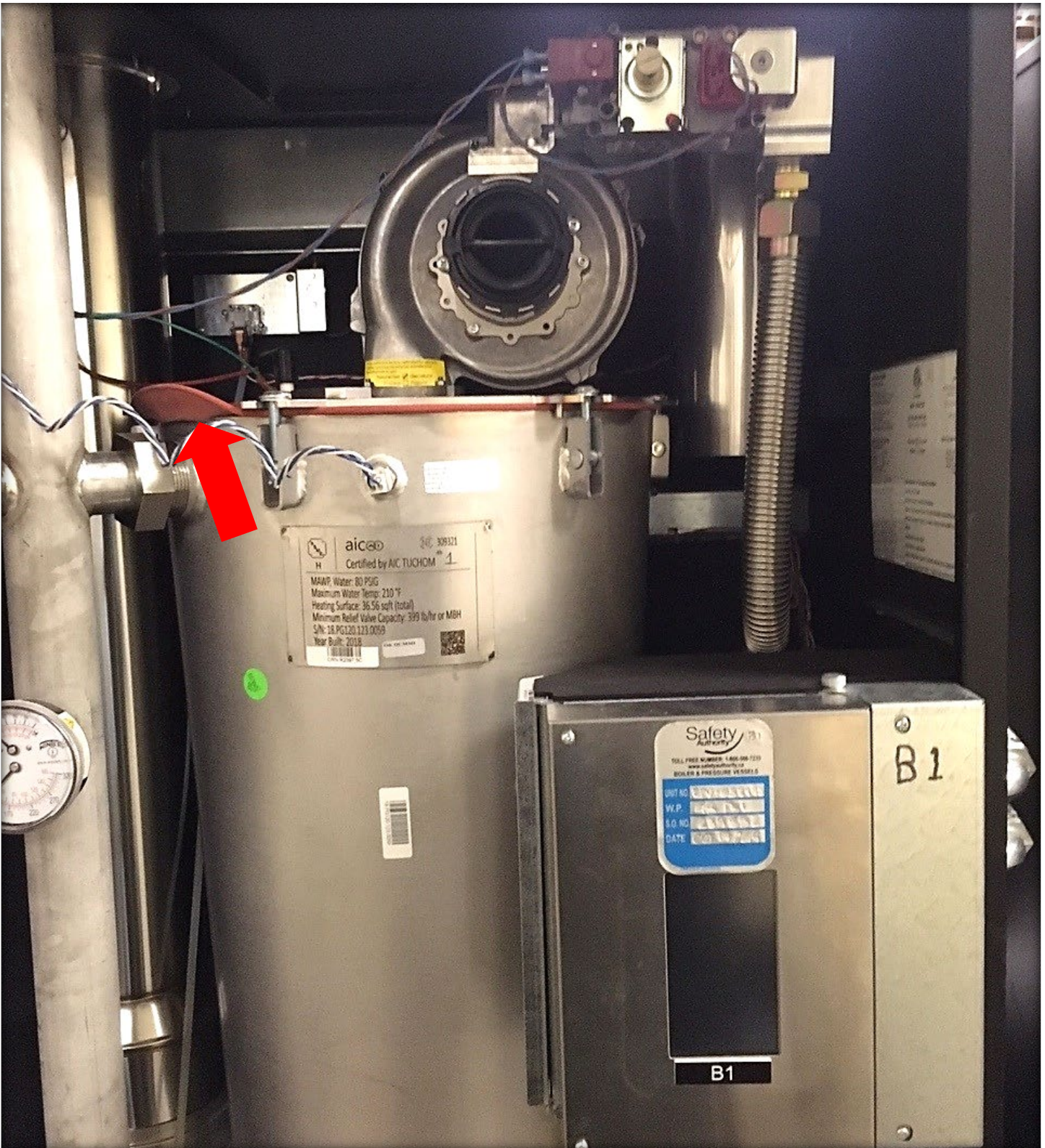
Image 6 – Pressure vessel gasket blown out from delayed ignition on Boiler 1 (example 2 of 4)
