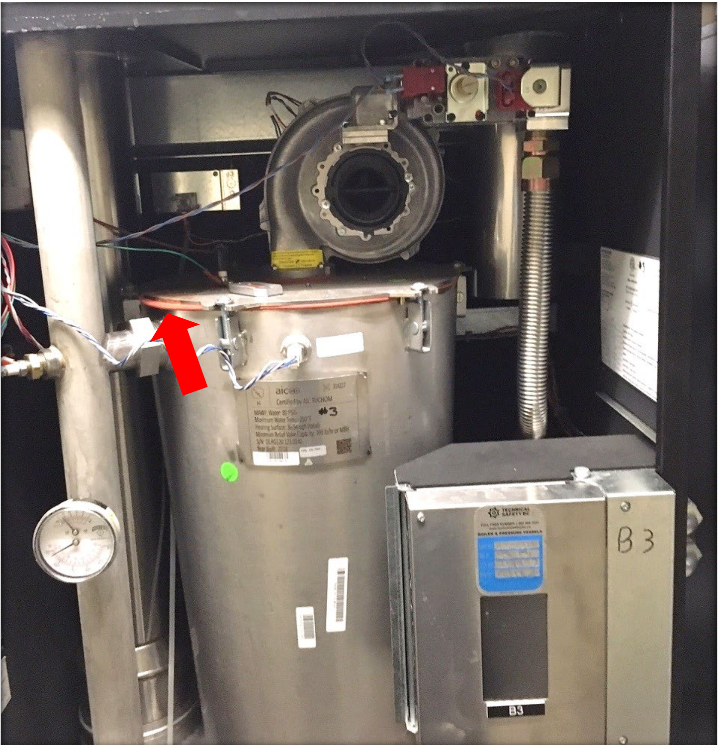
Image 8 – Pressure vessel gasket blown out from delayed ignition on Boiler 3 (example 4 of 4)
