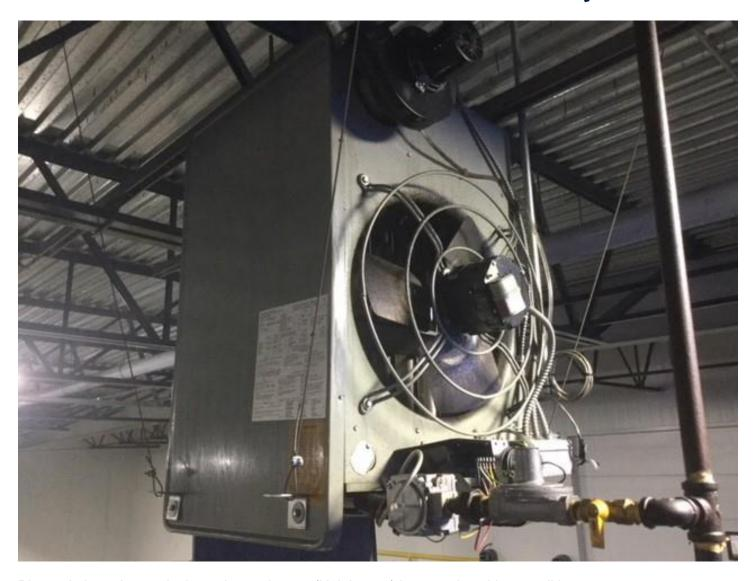
Pictured above is a typical warehouse heater (Unit heater) in normal working condition.
