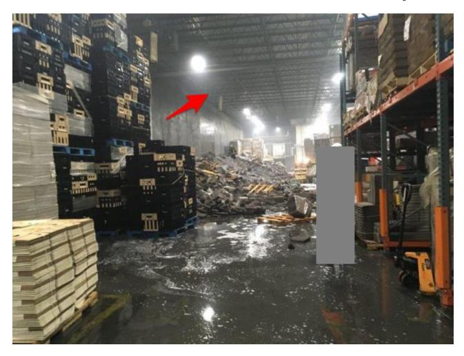
Fire damaged combustibles laying in a pile. The red arrow points to the approximate location where the heater was hanging from the ceiling.
