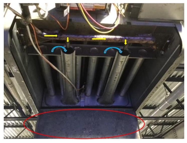
Looking up at the burners and flue passageways on a heater in good working condition.
