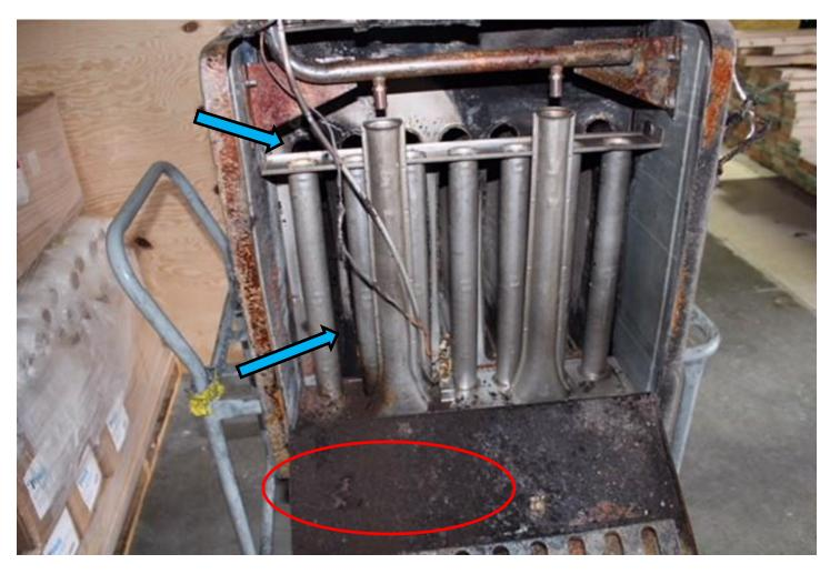
A view of the burners of the damaged heater. This heater was removed from site and is currently laying on it's side on a dolly for easy inspection.
