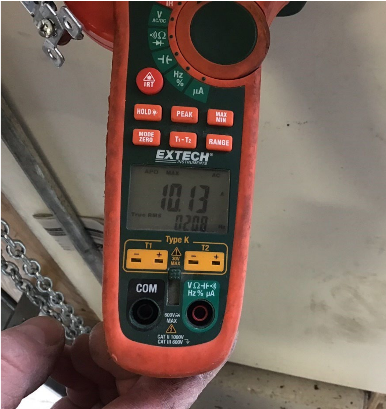
Image 3 - Load test: 10.13-amps
