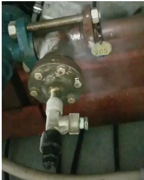
Fig. 3: Strainer cover plate and flange (picture taken during leak investigation)
