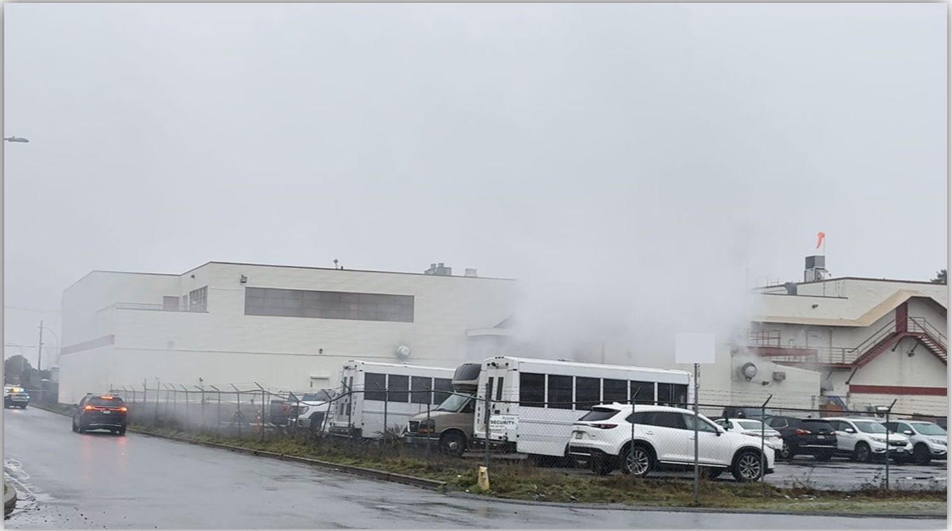
Image 2 – Screenshot of a video showing the rear of building and white fog of released ammonia from refrigeration compressor relief valve stack. Road closed by responding emergency services.
