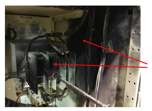
There is minor arc damage to the inside of the switch.
