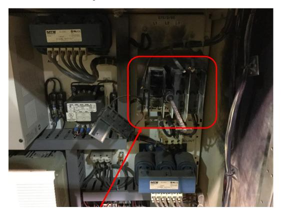
The fuse holder that the electrician was going to remove
