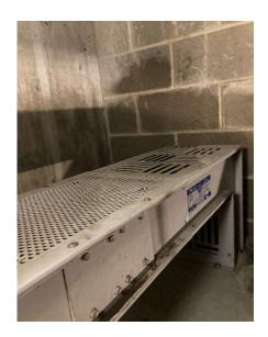
Photo group 5 – bus duct entering central distribution panel below bus duct
