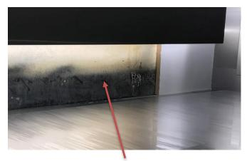
Photo 3: Close up view of where the panel had fallen out
