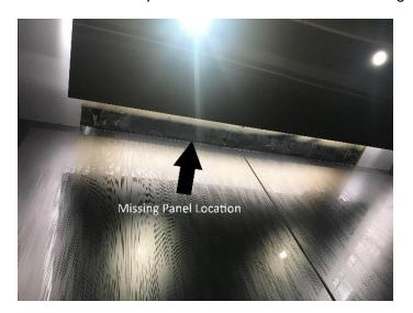
Photo 2: Location on the ceiling where the panel had fallen out of
