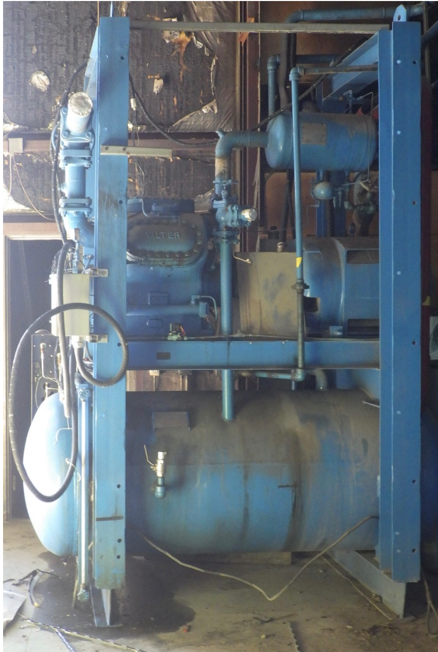
Figure 1: Refrigeration skid containing receiver, compressor, compressor motor, and oil separator
