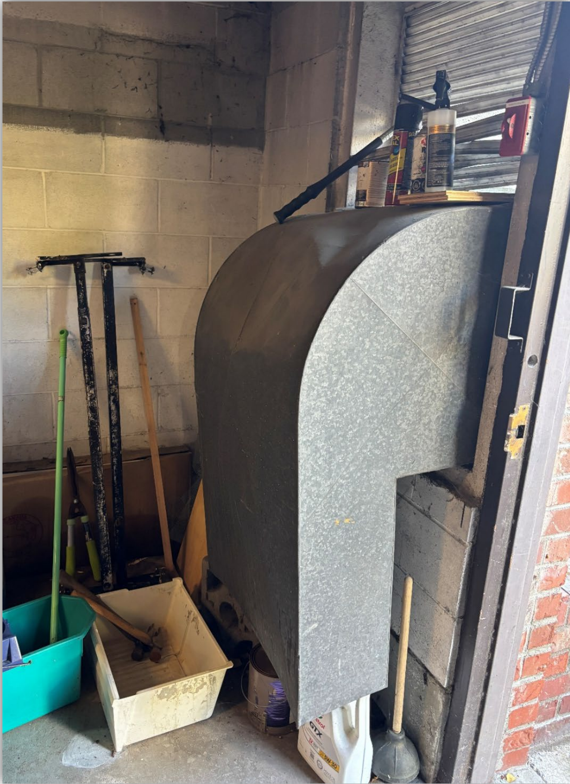
Image 9 – Combustion and ventilation air openings for mechanical room.
