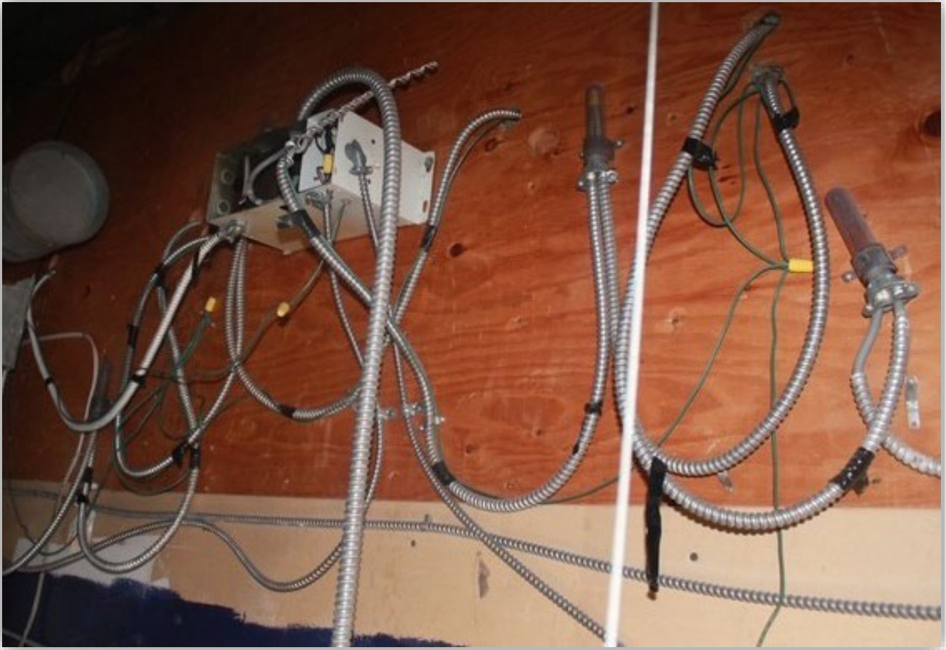
Image 3A – Conductive wiring not terminated.
