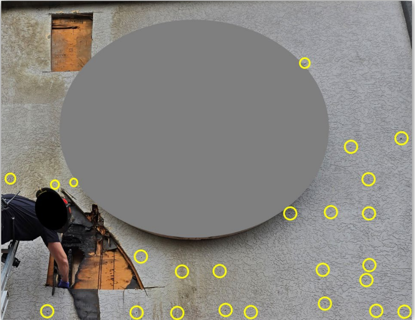
Image 2 – The circled items throughout the image shows some of the screw holes that were left in the envelope from several years prior when neon sign was removed.
