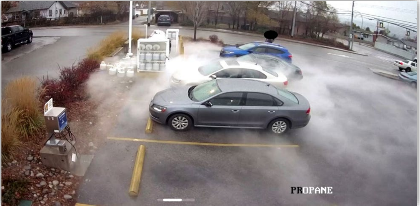
Image 4 - Video still image of incident showing extent of plume just before propane was shut down.
