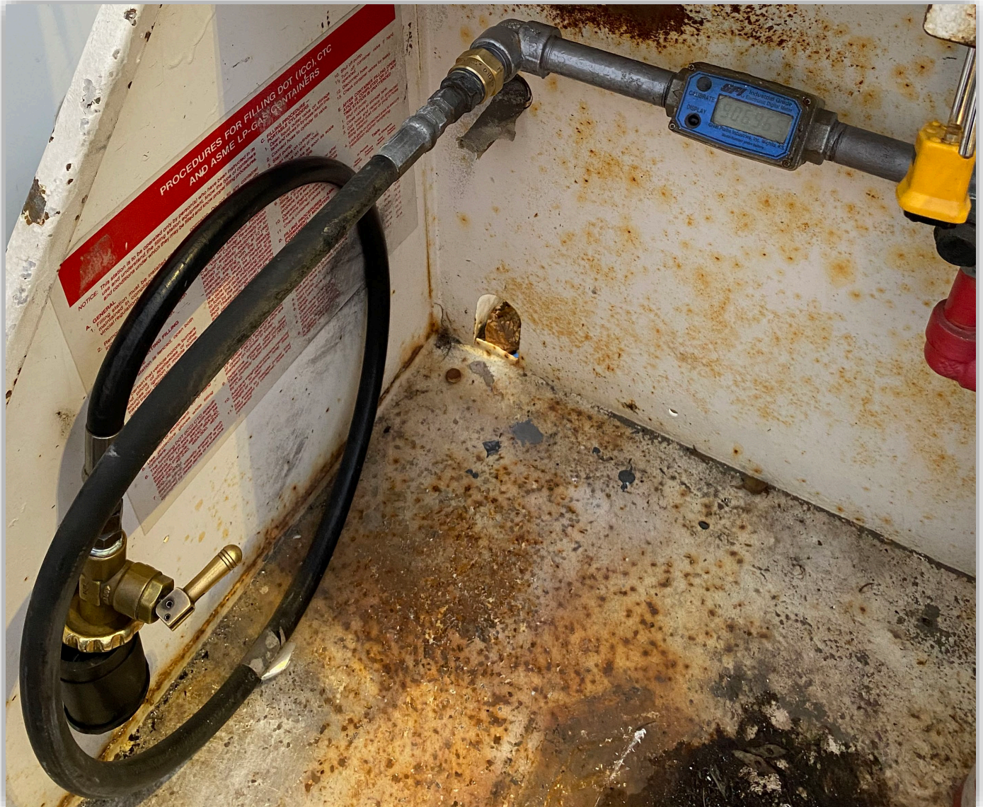
Image 9 - The propane dispenser once non-compliances were corrected, and excess flow valve and nozzle holder were installed.
