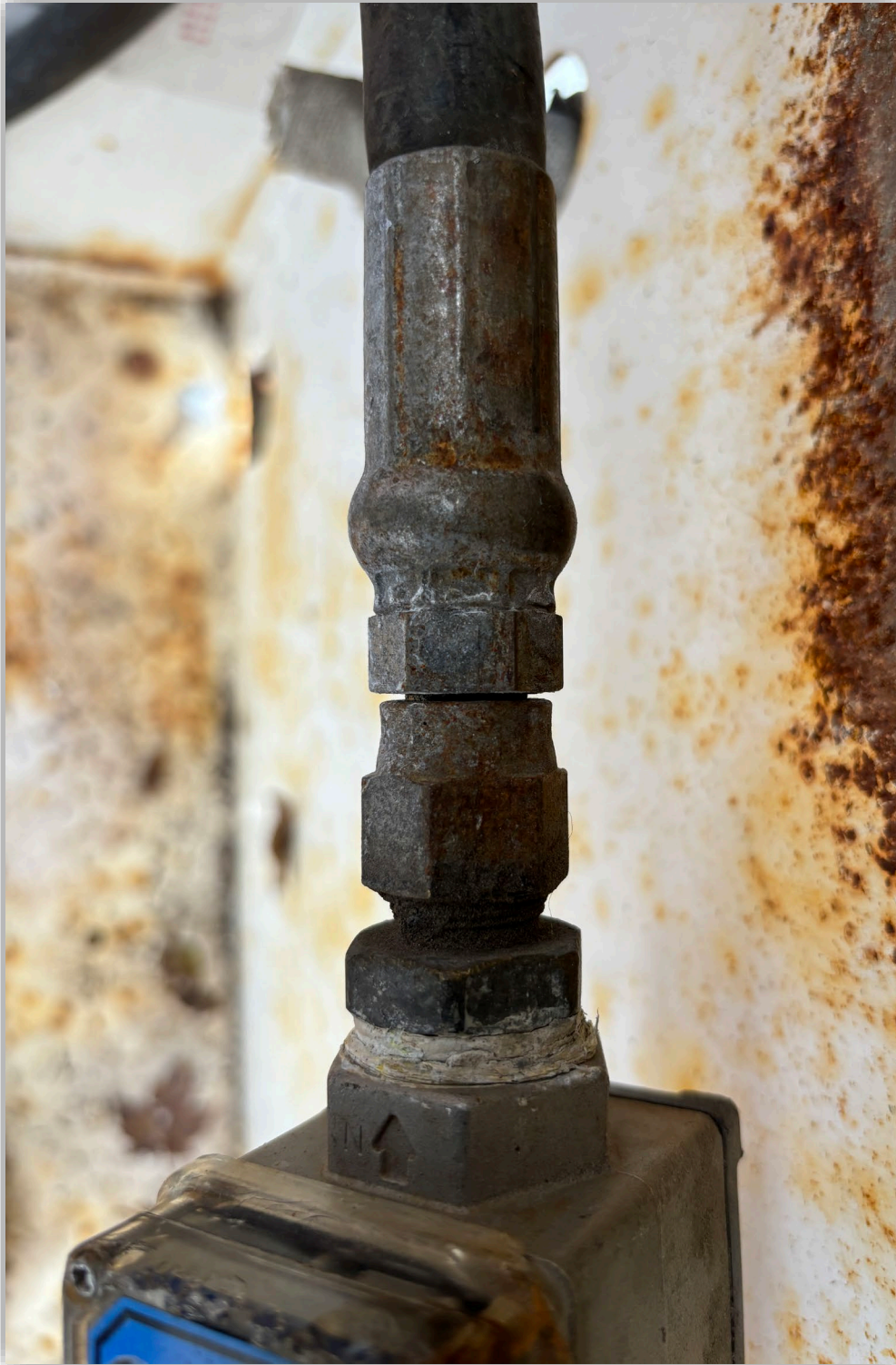
Image 6 - The one end of propane dispensing hose without excess flow valve.
