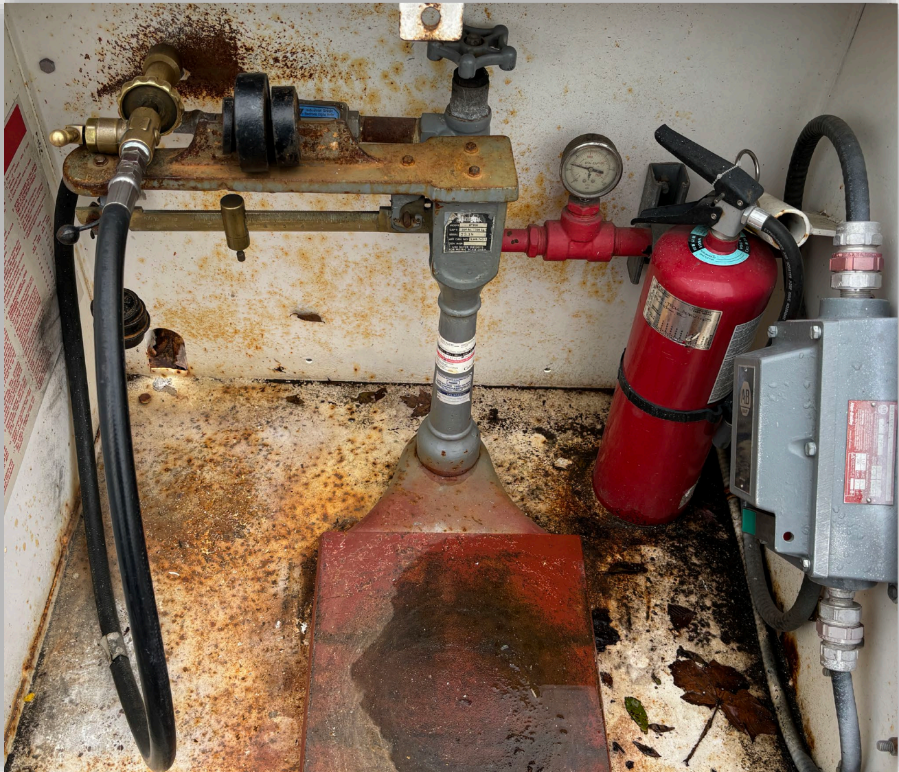
Image 5 - Propane dispenser showing how the cylinder fill nozzle was set down on day of incident.
