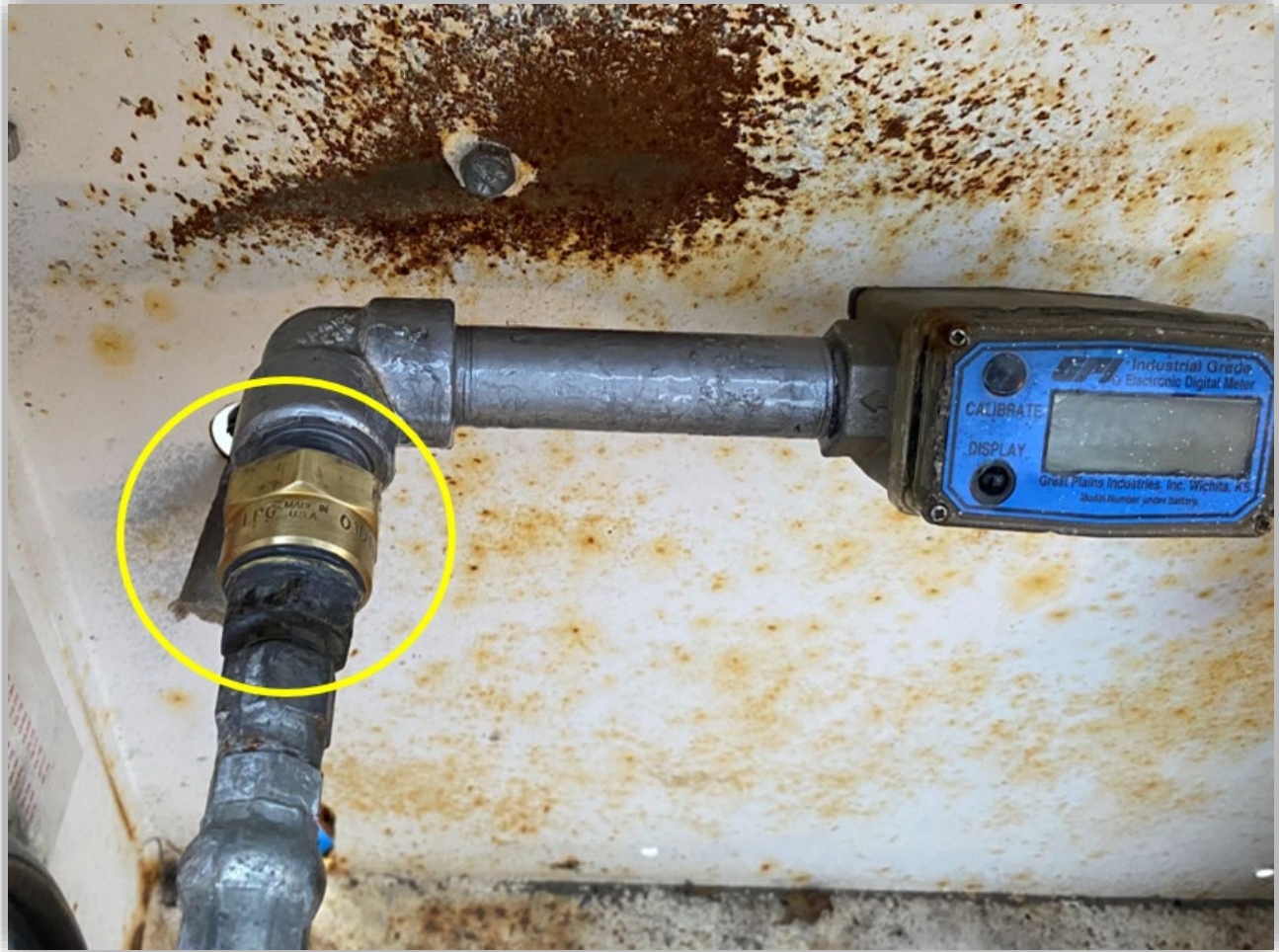
Image 8 - The propane dispenser after non-compliances were corrected. [Circle] Newly installed excess flow valve after the incident.
