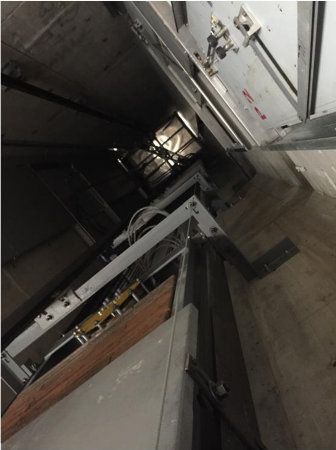
Photo #7- Photo show car resting in the overhead while the counterweight rests on the buffer.
