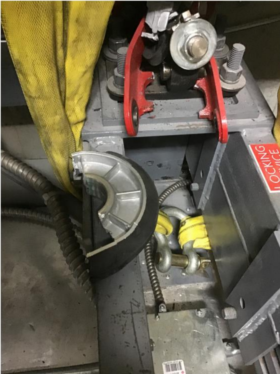
Photo #6 – Damaged roller guides on top of car
