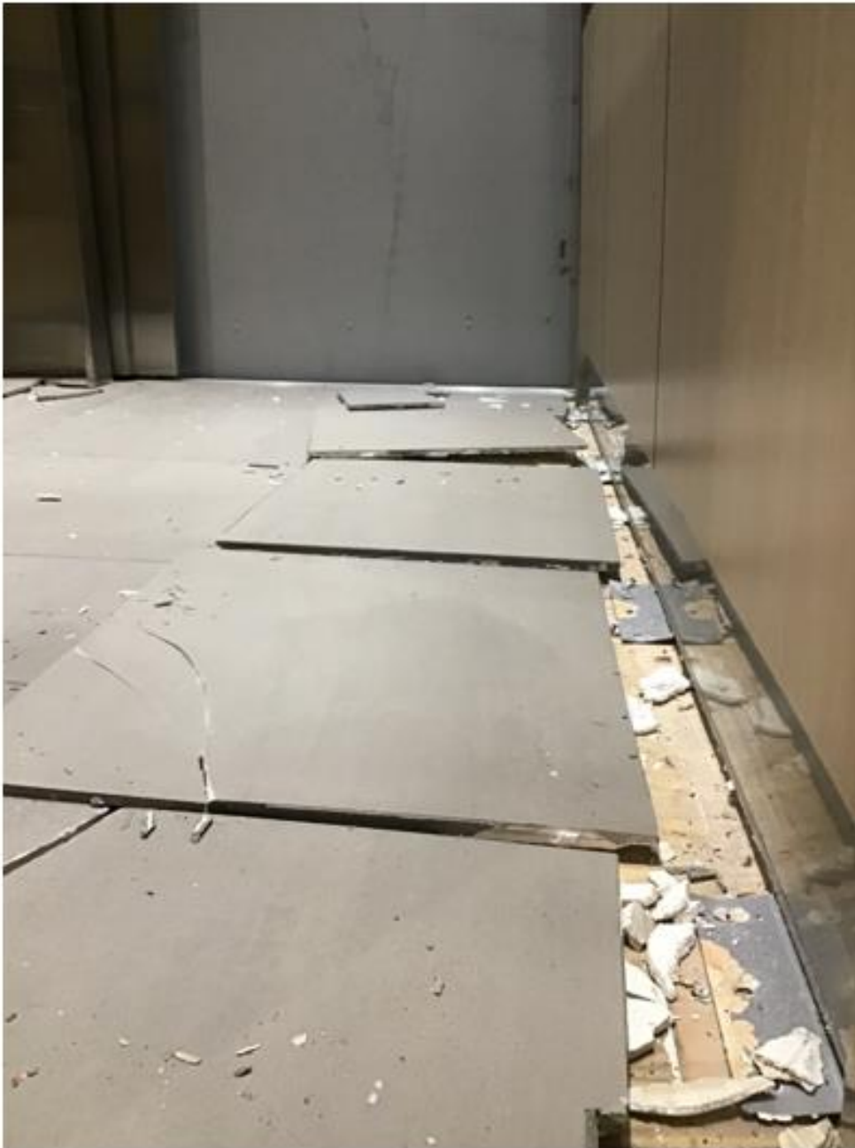
Photo #5 - Damaged floor tiles from impact
