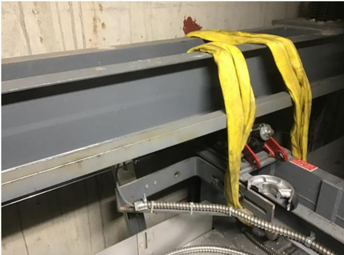
Photo #4 - This pic from the top of the car shows the hitch beam that it came into contact with. Rollers were damaged upon impact.
