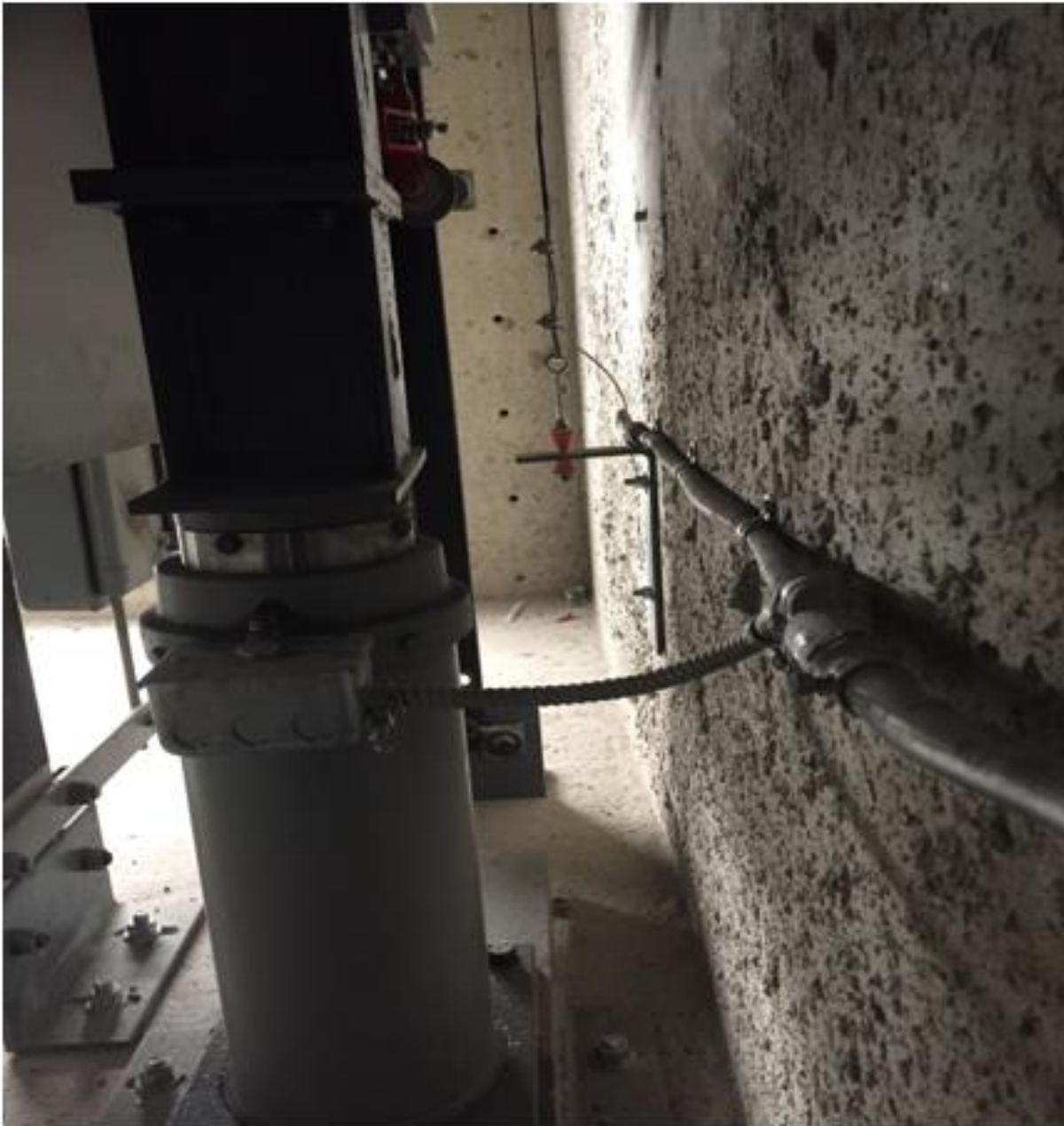
Photo #9 - Picture shows a compressed counterweight buffer.
