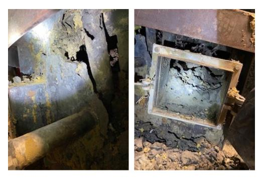
Outer shell steel melted away.
