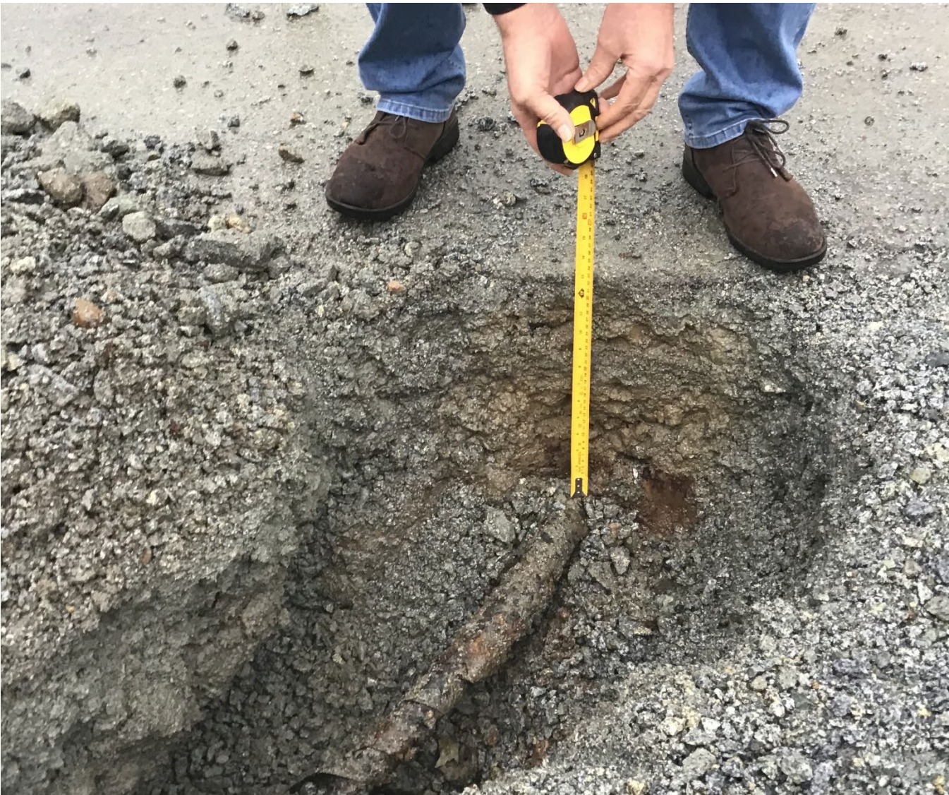
Image 3 - The measuring tape shows the high voltage cable is only buried 30cm below finished grade at roadway and there is no caution tape buried in earth above the cable to warn excavator of buried electrical equipment cable. This cable is required to be buried at least 100cm below finished grade surface and must have a cautionary marker tape or other markings to warn excavators of buried electrical equipment.
