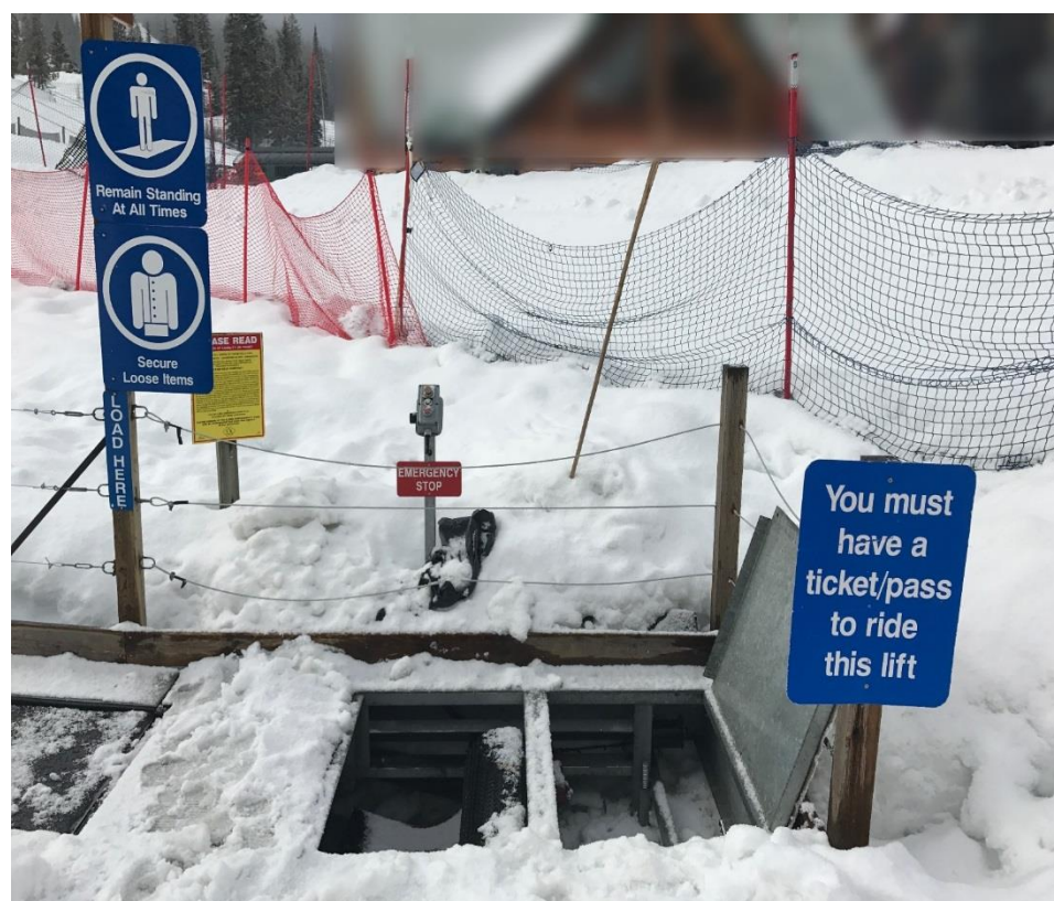
Figure 7: View of tail unit and drum. Snow covered and slippery surfaces. Tripping hazards.
