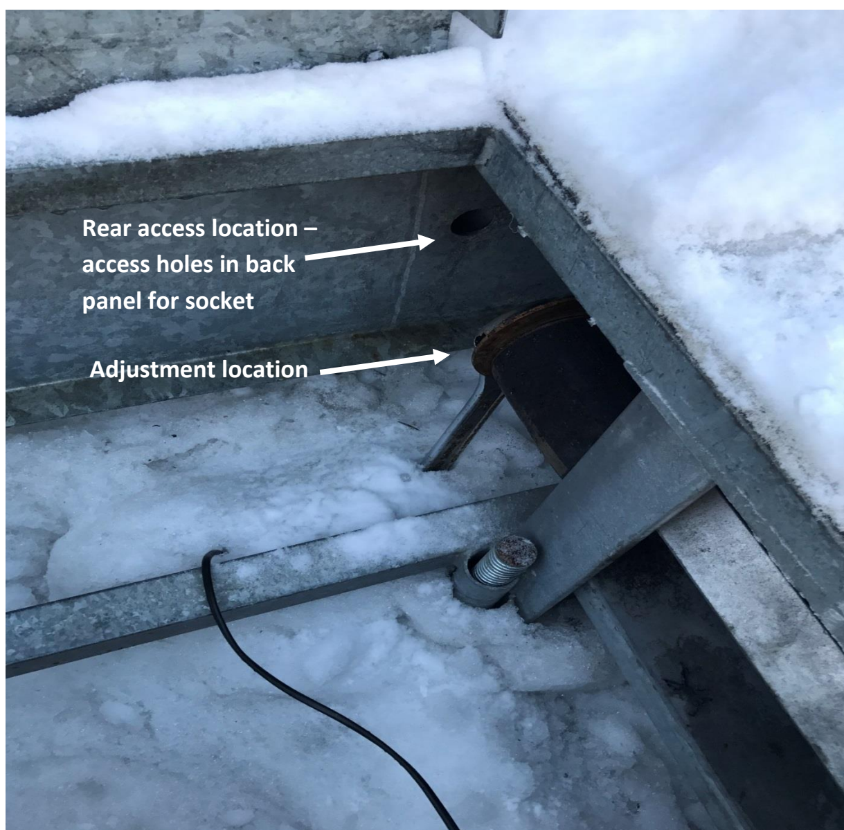
Figure 3: Adjustment rod with tension spring.
