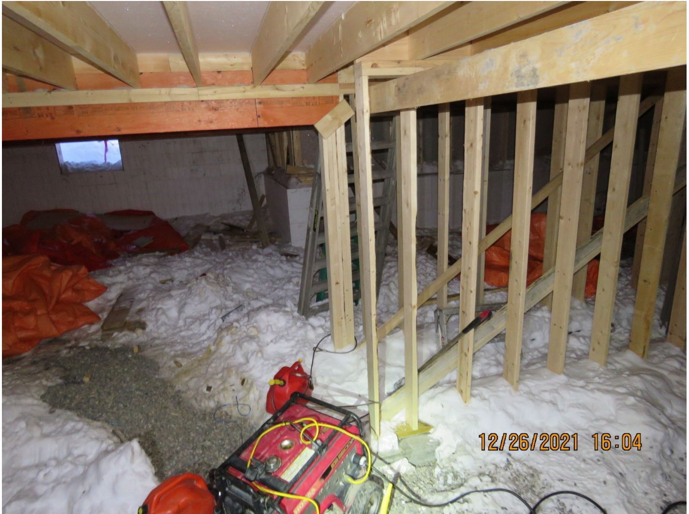
Image 2 – Basement of house under construction. Generator (bottom) with fuel cap off and nozzle readied on gas can.
