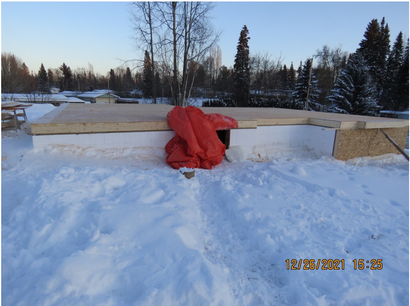
Image 1 – Insulated concrete block formed basement walls with plywood subfloor. Single point of entrance with orange tarp.
