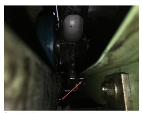
Step hold down track and step up lift tab.
