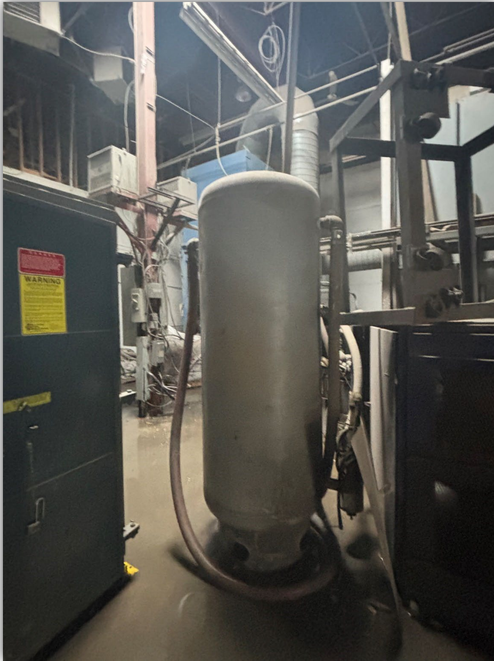
Image 3 - Supply Tank 1 with compressor on the right.
