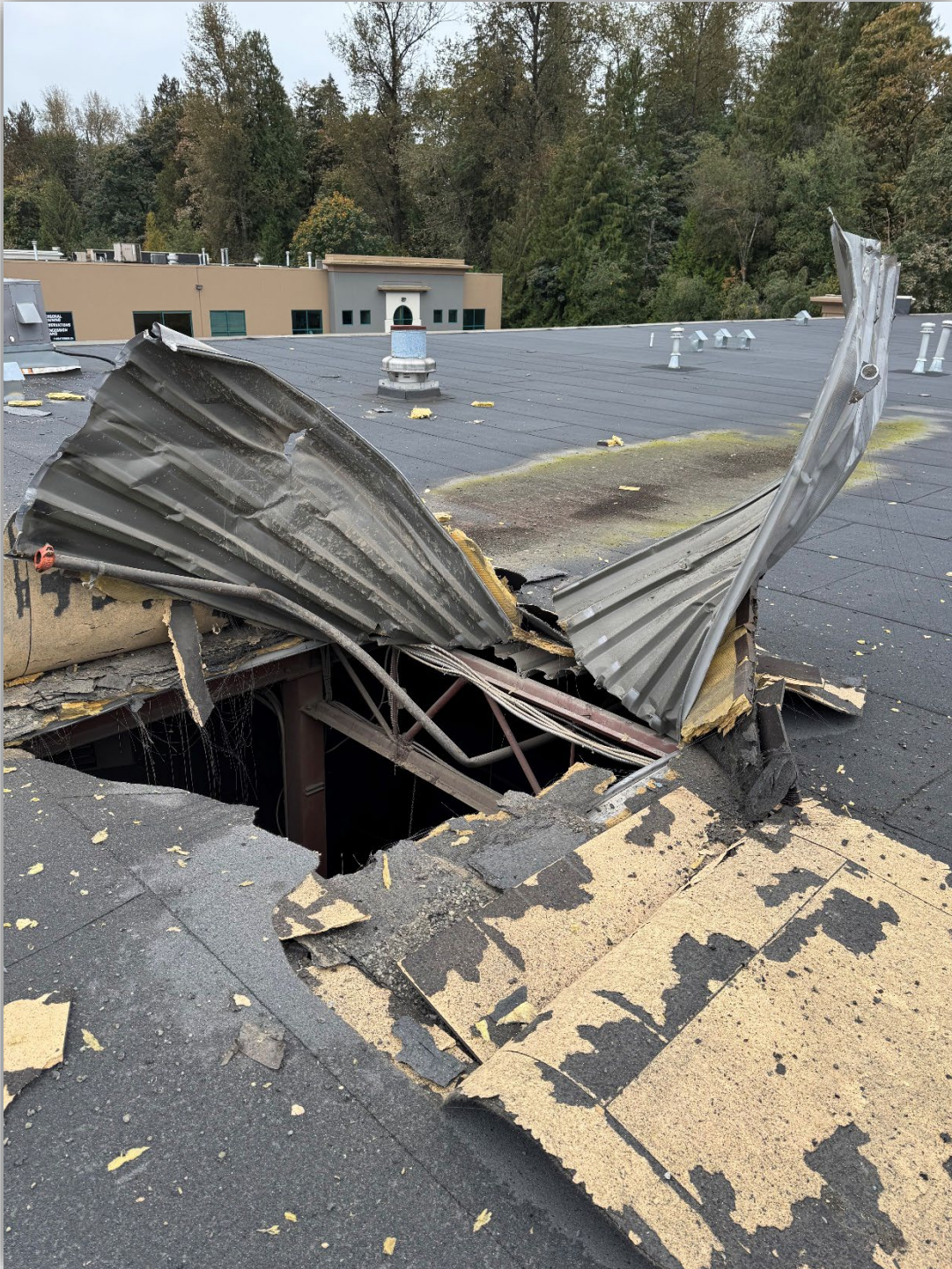
Image 9 - Hole in roof caused by tank failure, external view.
