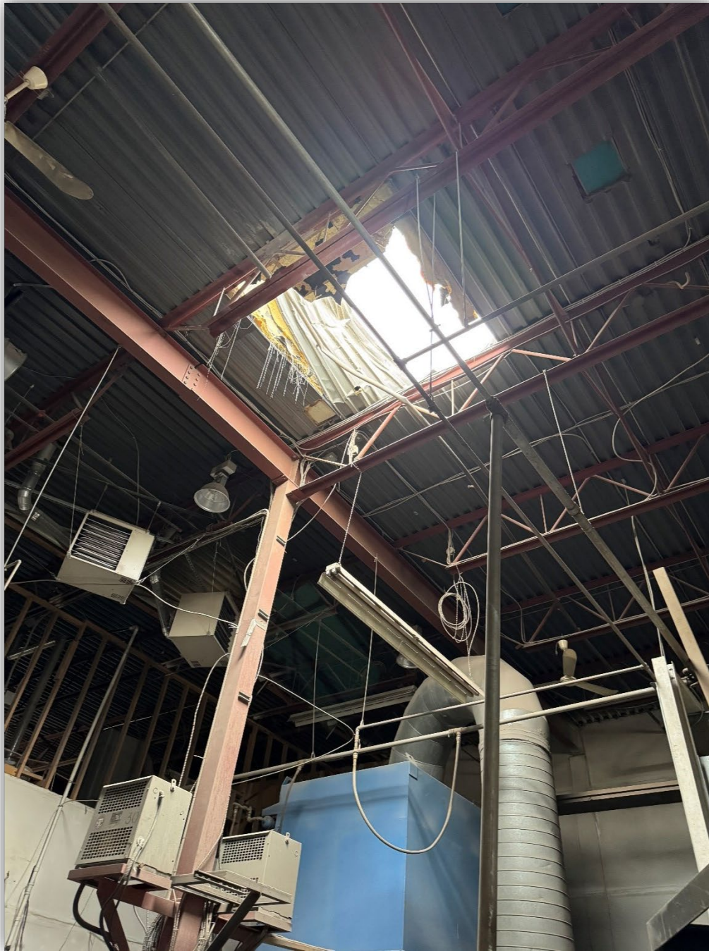
Image 8 - Hole in roof caused by tank failure.
