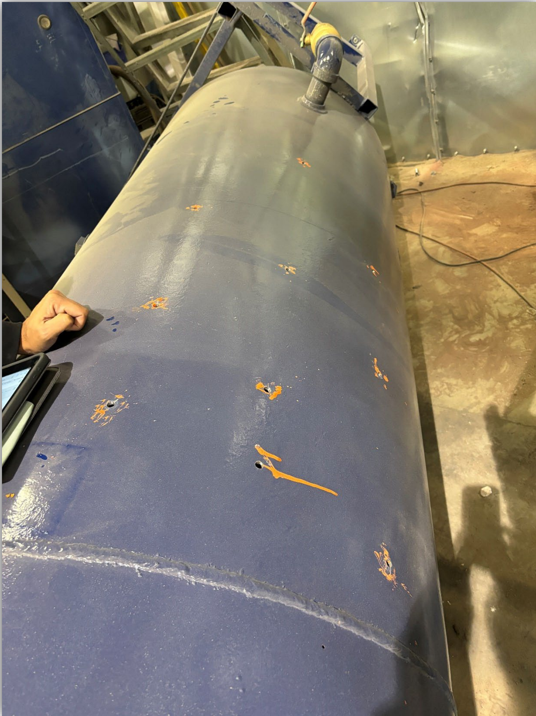
Image 23 - Supply Tank 3 – owner drilled holes in Supply Tank 3 so it could not be returned to service.
