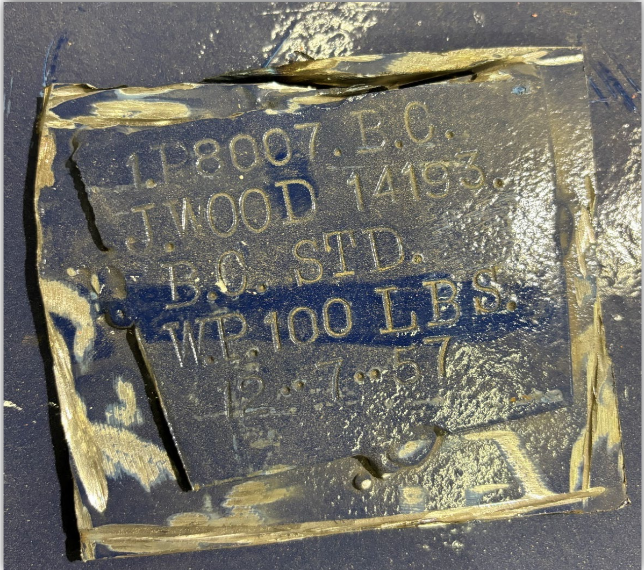
Image 22 - Supply Tank 3: nameplate cut out.
