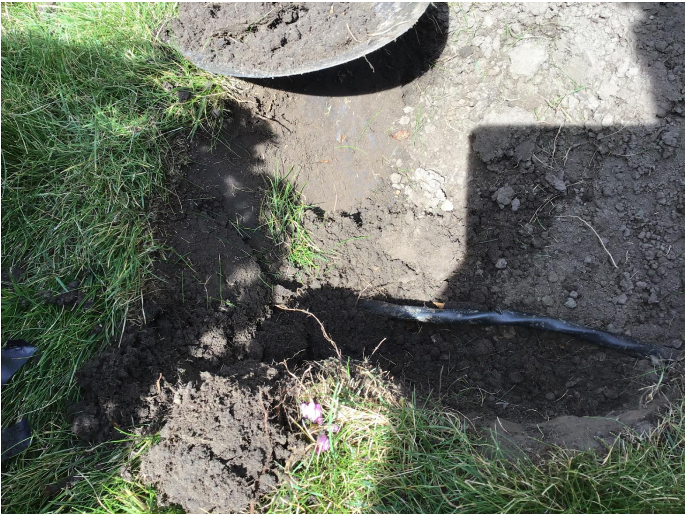
Direct buried wire at shallow depth
