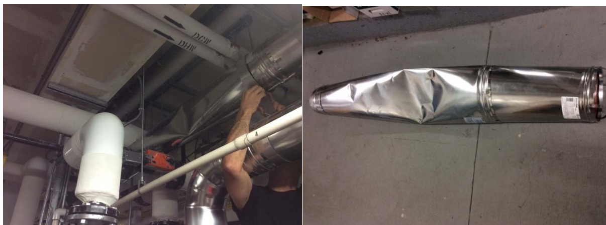
Collapsed venting on horizontal run
