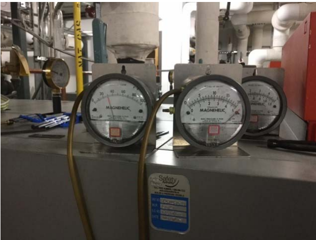
Lock up pressure test (right hand side) downstream of regulator, upstream of gas inlet to the boiler
