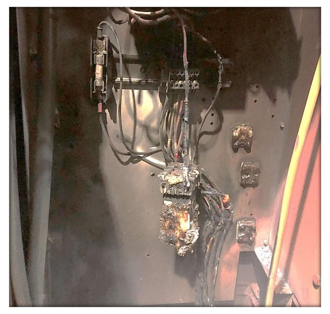
Figure: 1 – Internal components, floating relay, and damage.
