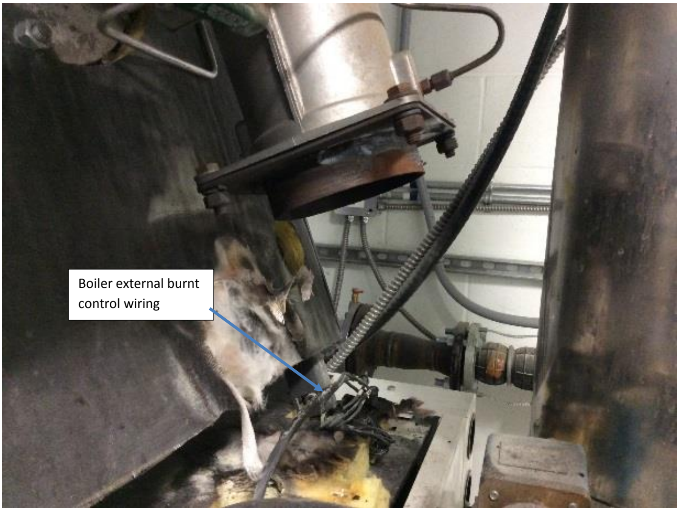
Photo 3: Burnt wiring exterior top end
