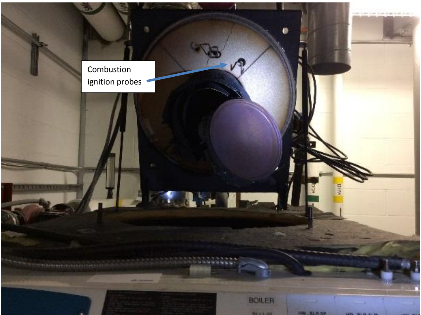
Photo 2: Ignition probes - top end
