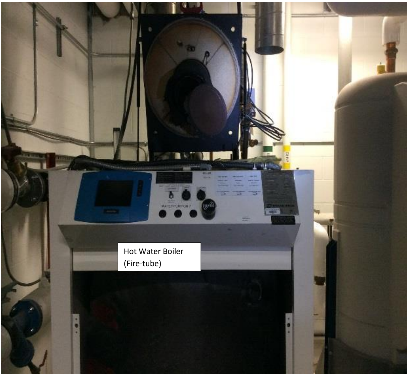
Photo 4: HW Boiler front & open combustion area
