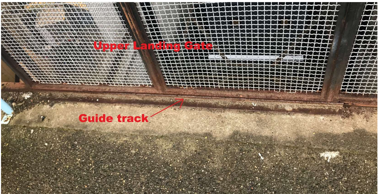
Photo 2 – Bottom of upper landing gate
