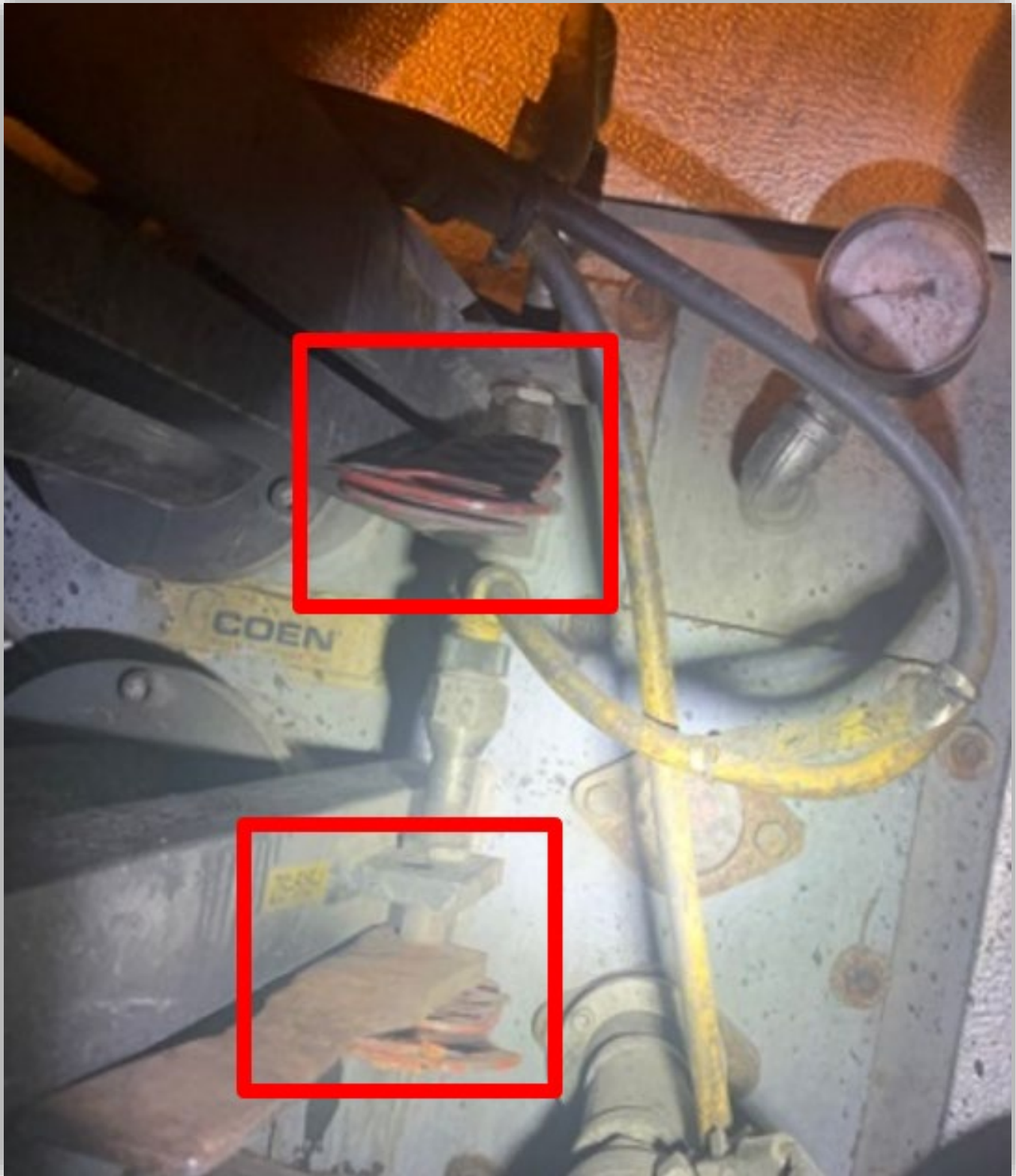
Image 3 – Shims used to bypass the safety limit switches.
