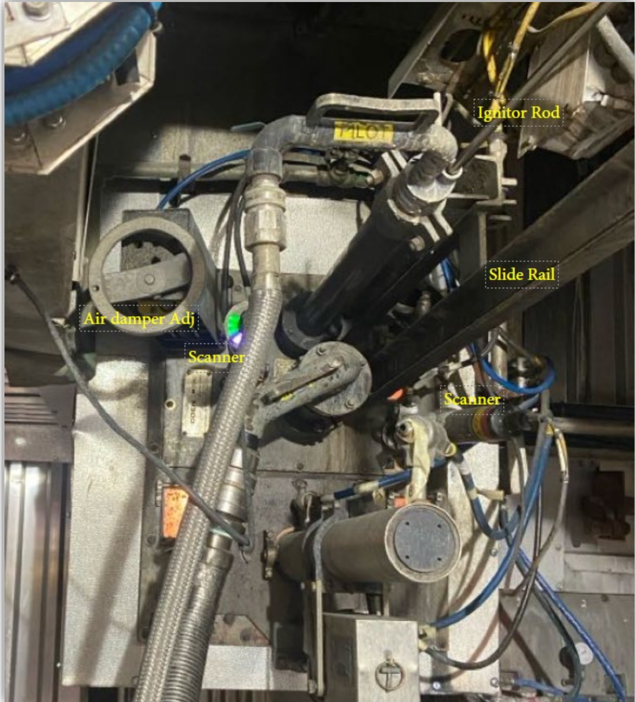
Image 6 – Burner assembly.
