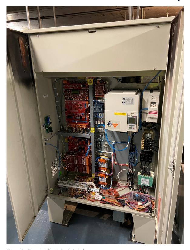
Figure 7 – Repaired Controller (Interior)
