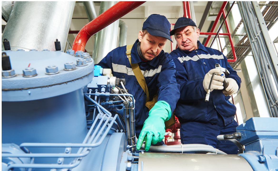
Inspections carried out by the asset owner
