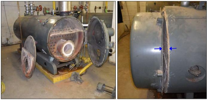
Photo 2: Boiler 2 front door open with burner removed (left), damaged rear door (right)
