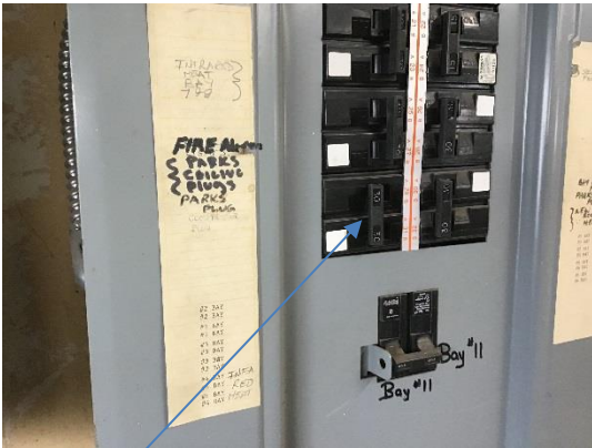
Photo#1: Branch circuit breaker
