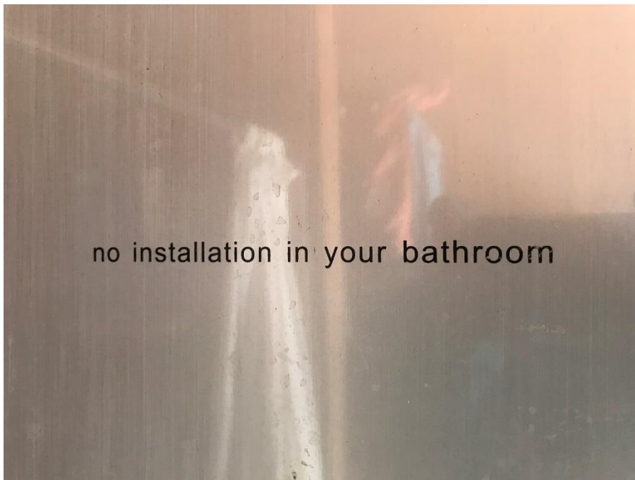
Image 8 (left) – Text (markings) on the front of the water heater cover reads “no installation in your bathroom”
