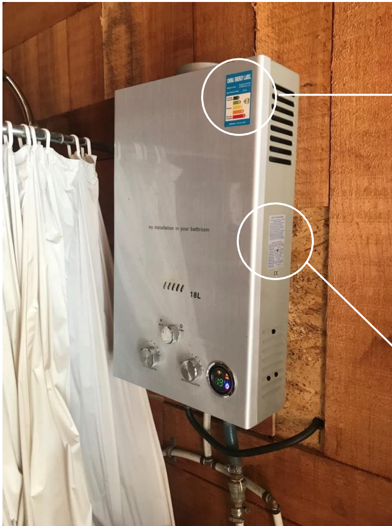
Image 4 (above) – Water heater installed inside shower building without flue vent piping
