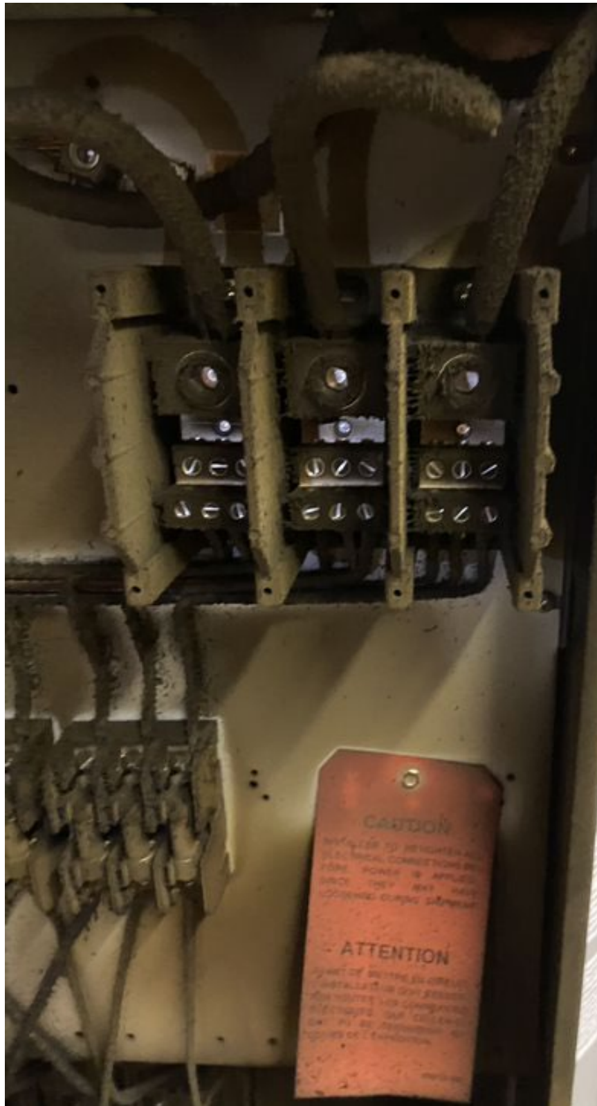
Photo 4 - Control block where incoming power terminates, located at the top of control module. Smoke and minor heat damage otherwise unaffected.
