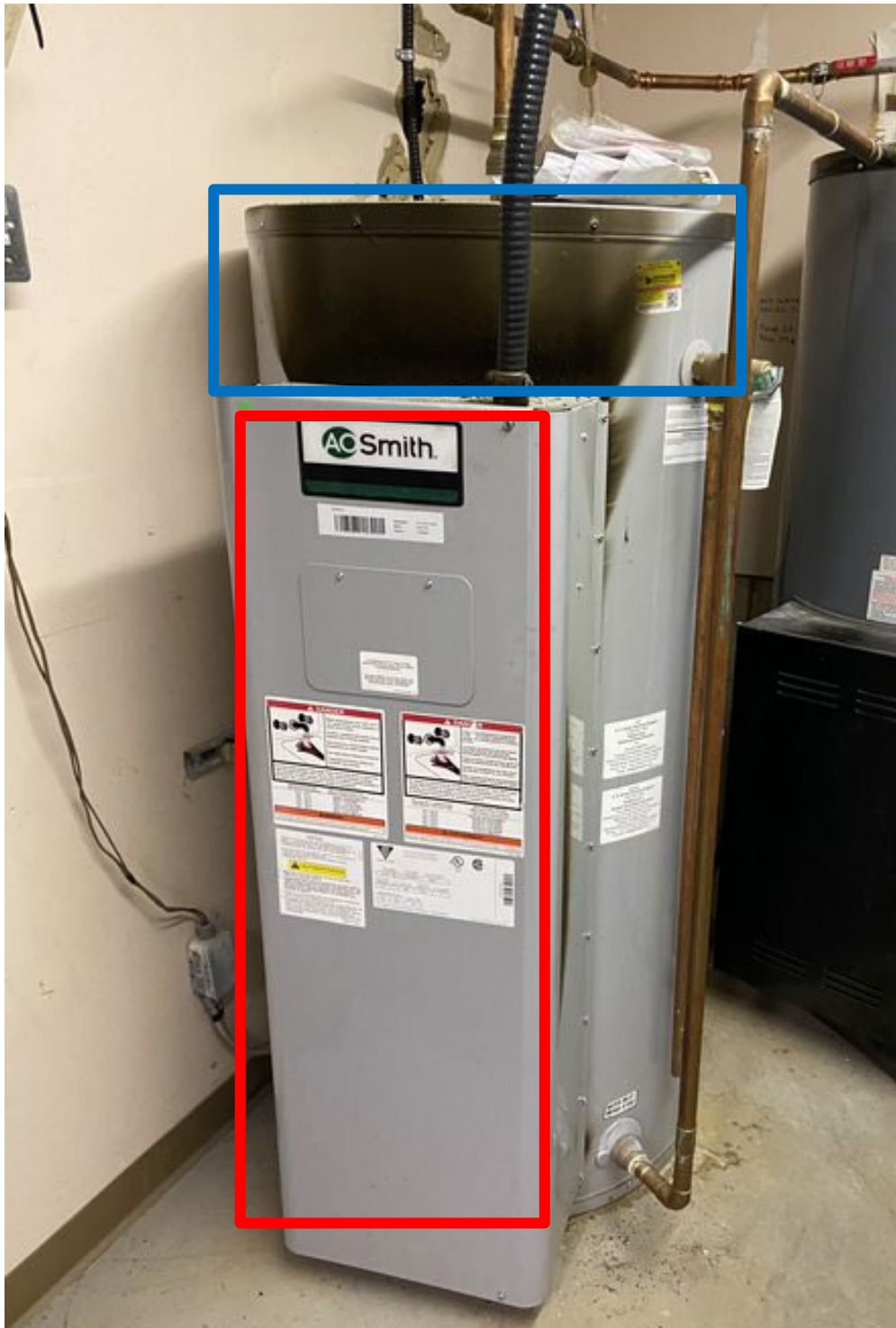
Photo 5 - HWT as found after fire. No clean up done. (BLUE) Smoke damage on the hot water tank above the control panel (RED).
