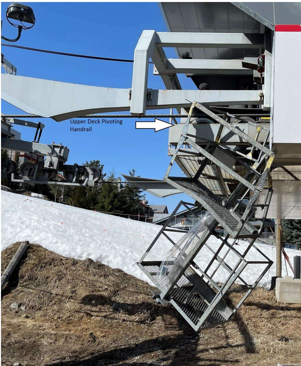
Photo of Entangled/Jammed Maintenance Carrier
