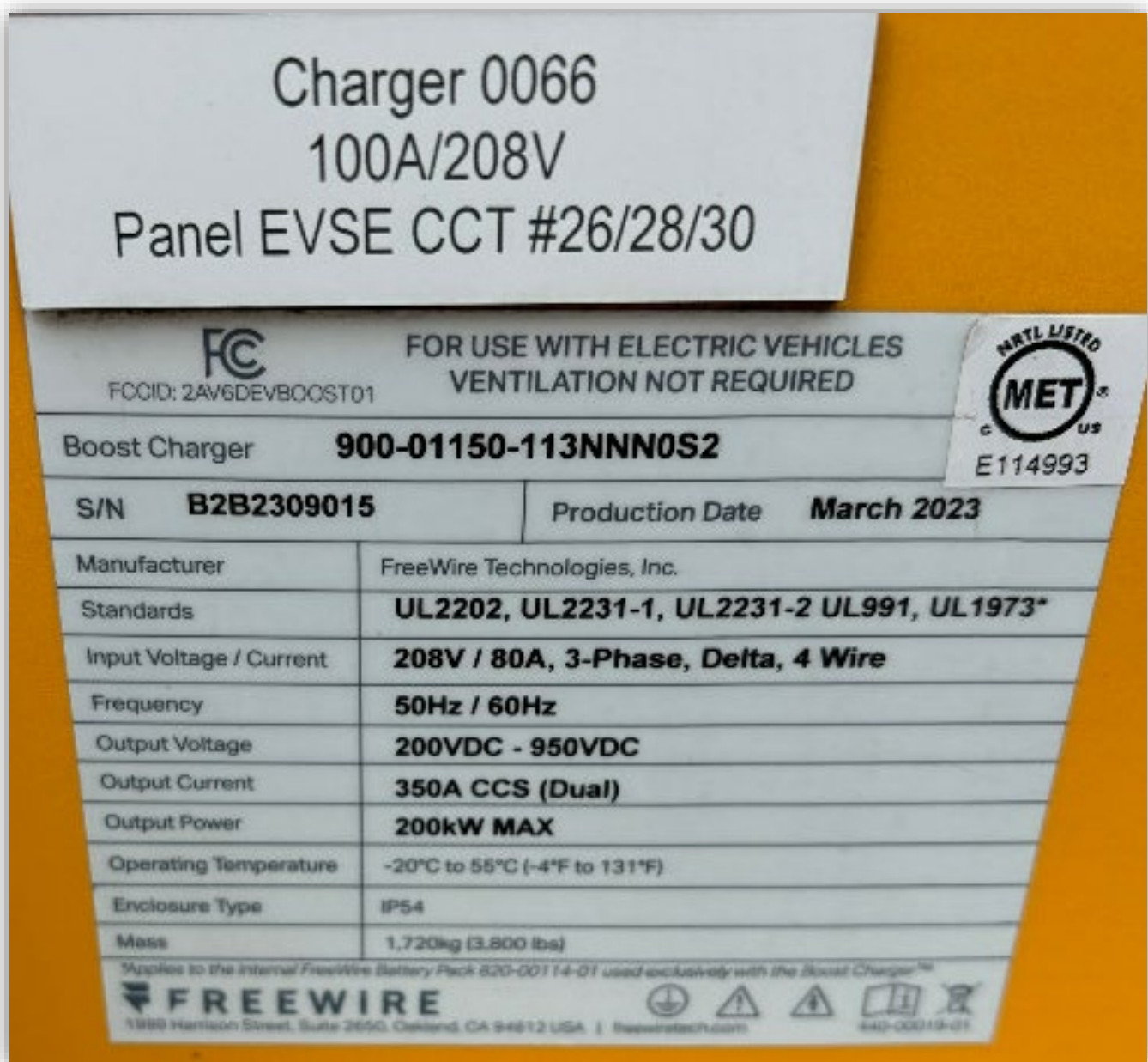
Image 5 – Data tag for the charging station showing 200kW max power output.
