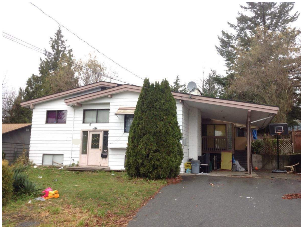
Photo 1: Front of the house where incident occurred.
