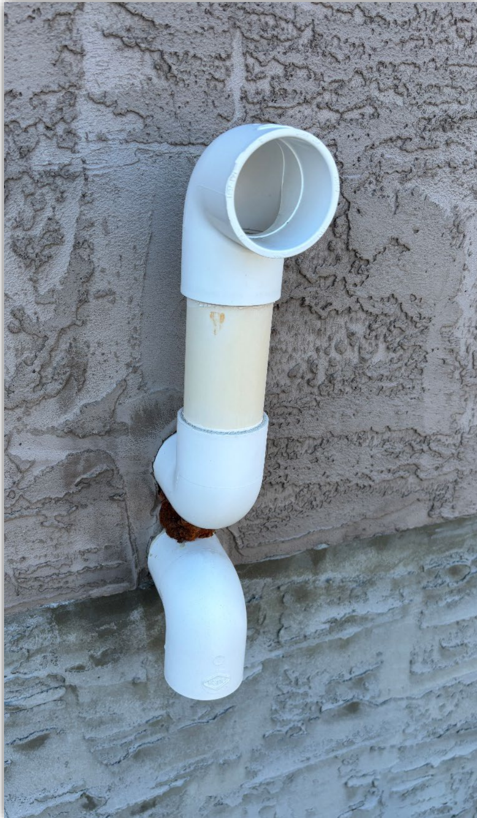
Image 9 – Furnace air intake (bottom) and vent pipe termination (top) on the outdoor wall of the home.
