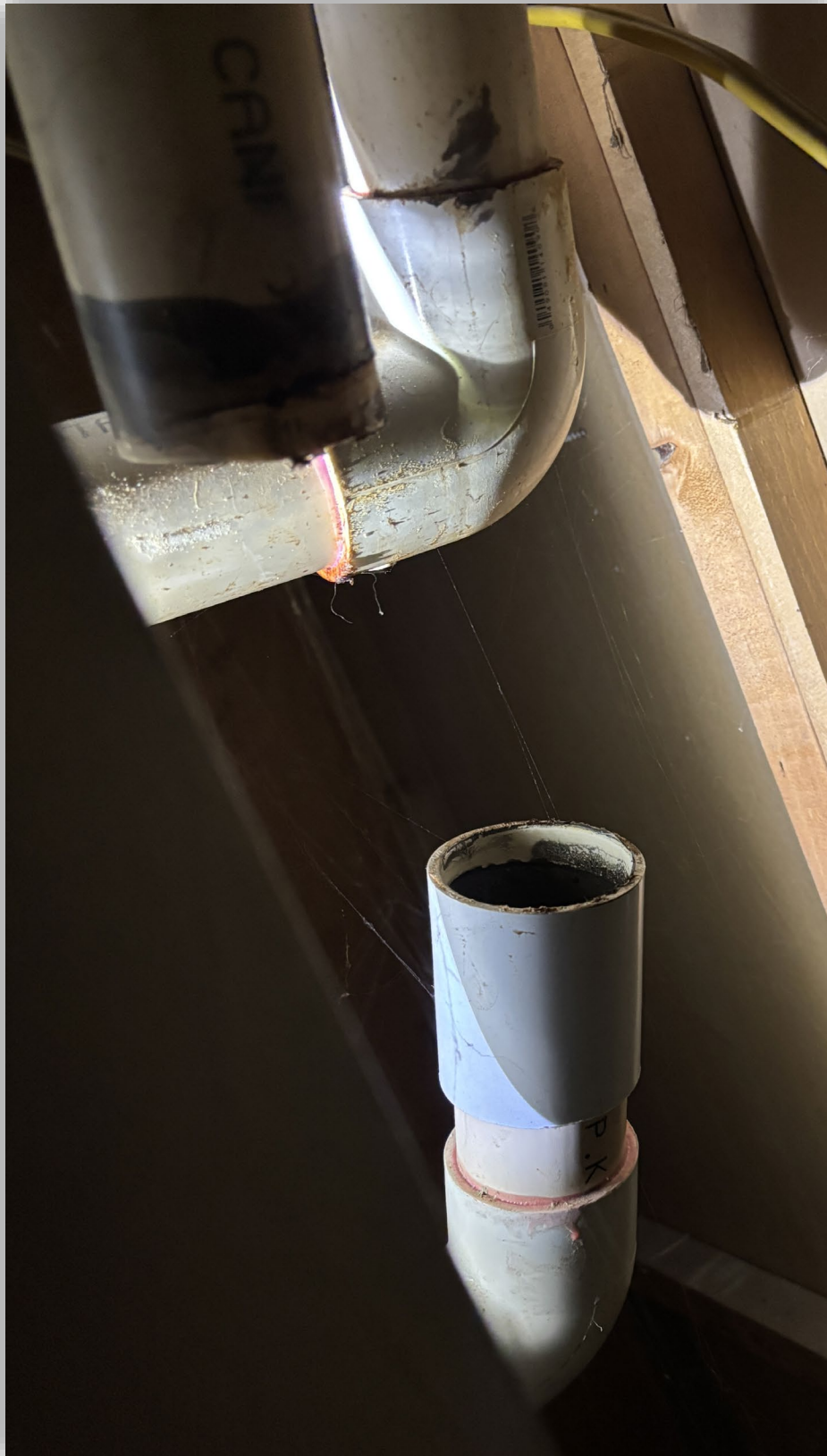
Image 7 – Disconnected flue vent pipe from other angle.
