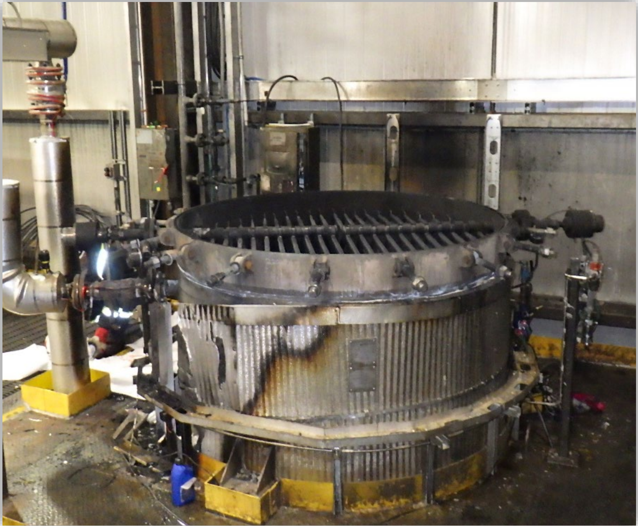
Image 2 - Fire damaged filter vessel with top cover removed.
