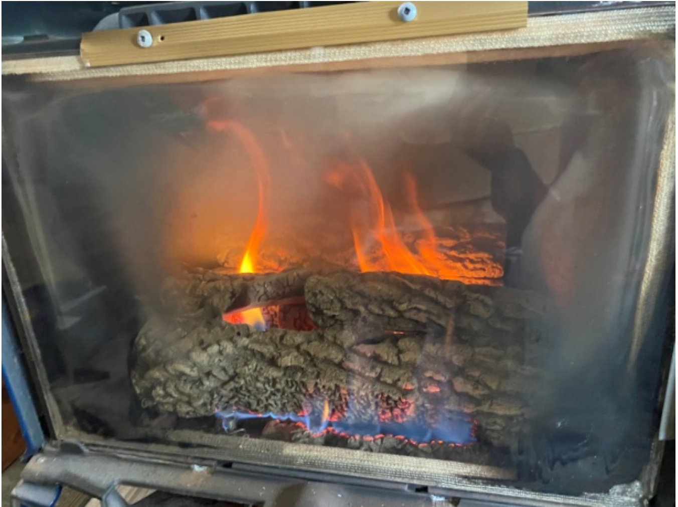
Photo 5 - Space heater burner on at high fire as found setting showing lazy yellow and orange flame indicating incomplete combustion.
