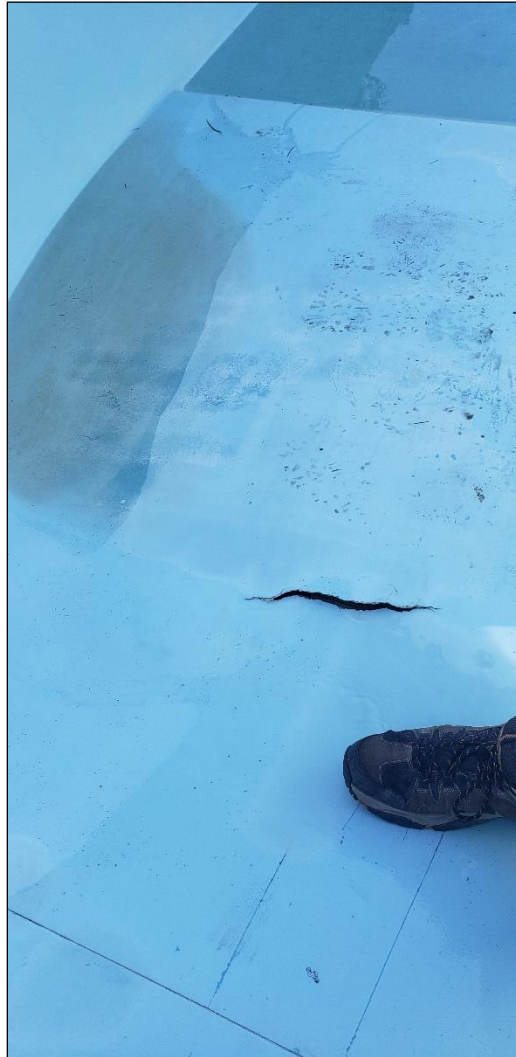
Figure 1 Overall view of transverse fracture in fiberglass slide.
